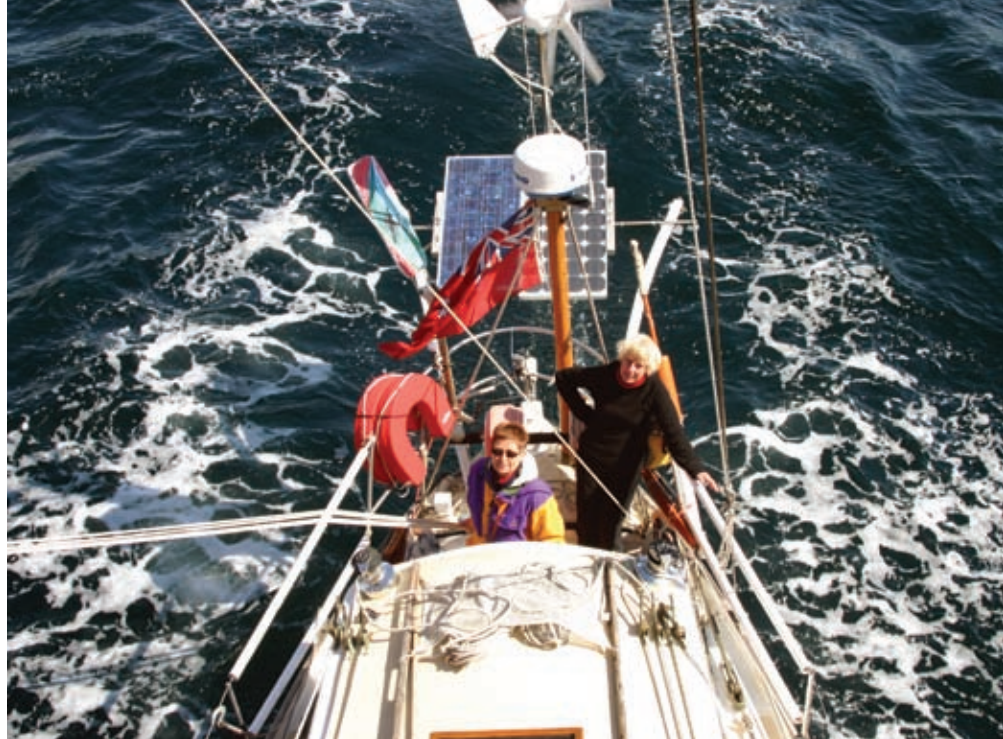
A wind generator and two solar panels (rated at a combined 120 watts) help keep up with charging demands for Balæna's house battery bank.
