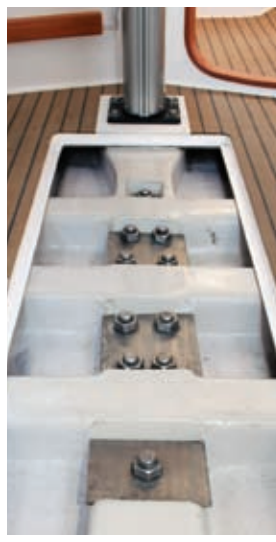
Keel bolts fasten through a large load-bearing plate recessed beneath the floors, part of a structural grid that absorbs sailing loads.
