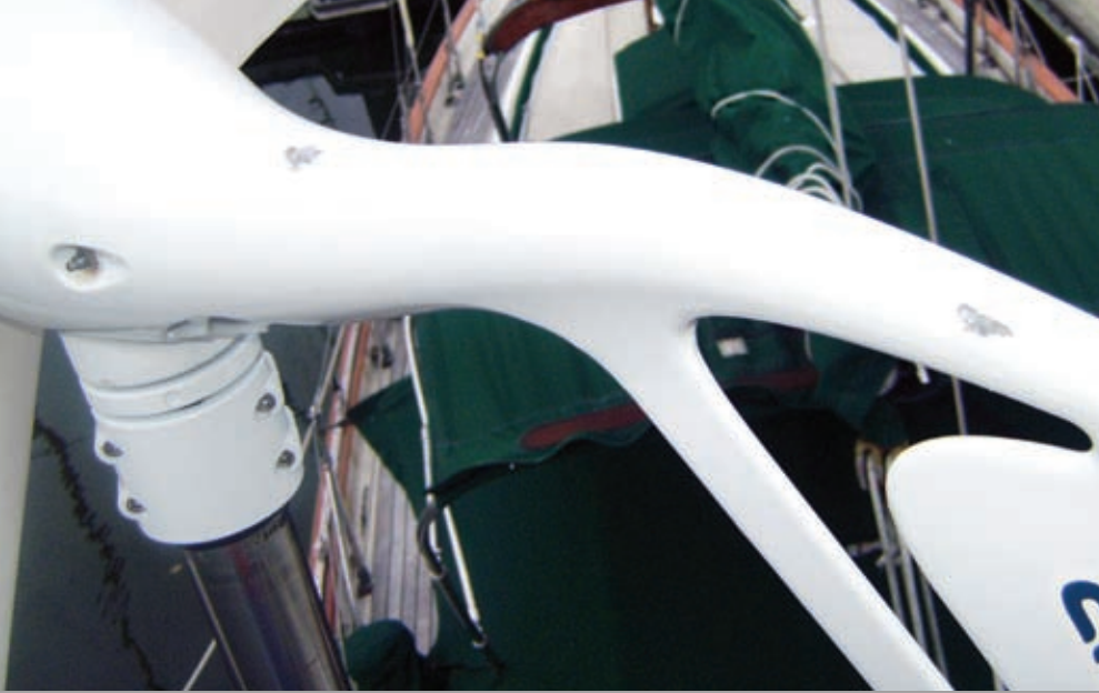
The powder coating on the aluminum body failed on the top of the tail fin assembly (above) and at the output adjustment screw (above, right).
